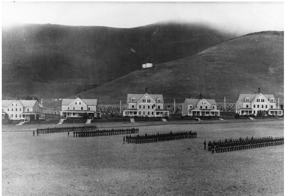
This is a 1906 photograph of the Fort Baker parade ground with Coast Artillery troops in formation and, around the perimeter, new married officers quarters built in the Colonial Revival tradition.
