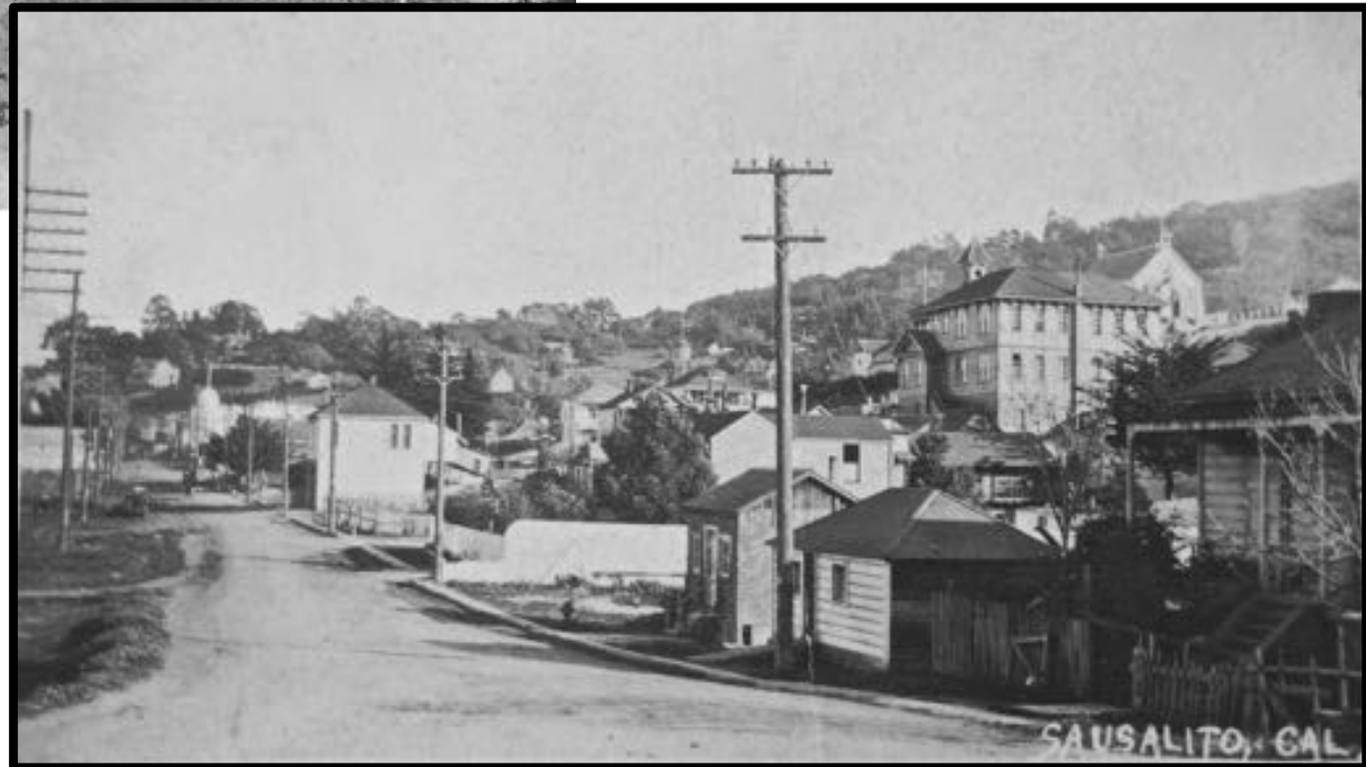
Pre-1920 – looking east on Napa Street and south on Caledonia from the Napa intersection
